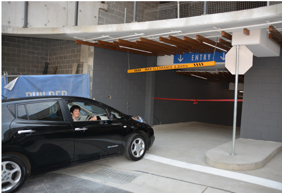
Mayor of Lane Cove Cllr Pam Palmer was the first to drive into the new car park at The Canopy on 6 December. The Mayor drove an electric vehicle highlighting the electric vehicle charging points available in the car park.
